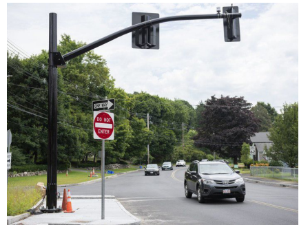
Black Intersection Mast Arms
