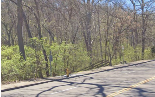
Current sidewalk conditions between Virginia Avenue and Highforest Lane along Colerain Avenue
